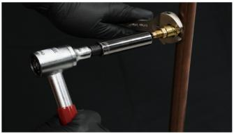
Use wrench to hold Seat in place to prevent applying torque to Seat braze while torquing Valve Core
